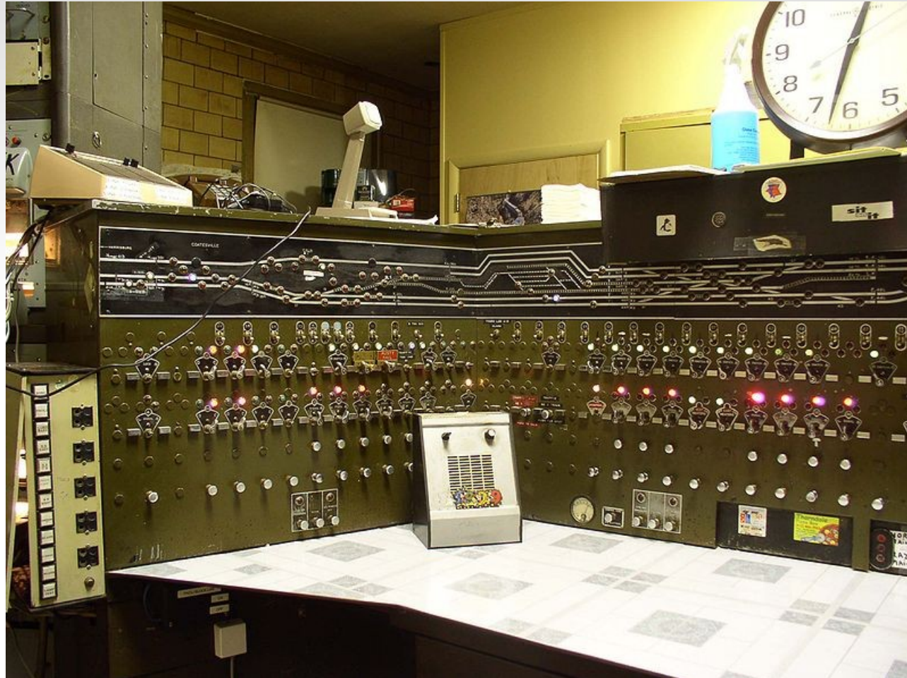
Active Union Switch and Signal CTC machine at Amtrak's THORN Tower.
